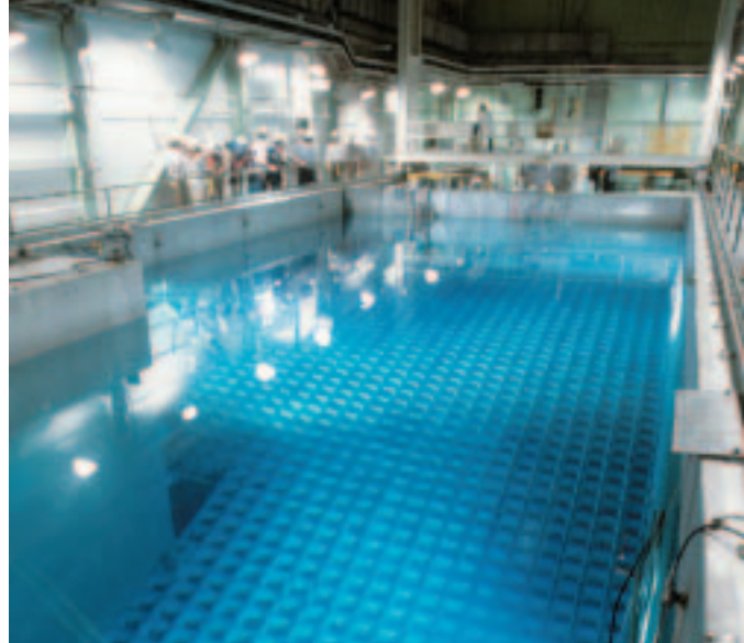
Figure 17 Spent nuclear fuel rods are placed underwater after they are removed from the reactor core. The water absorbs the nuclear radiation and prevents it from escaping into the environment.
