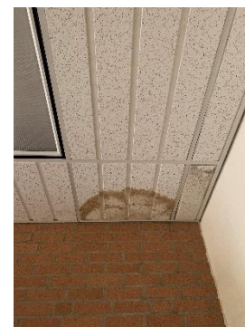
LEAKING/ STAINING AT JOINT OF NEW ADDITION
