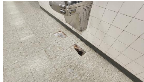
MISSING FLOOR FINISHES
