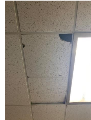
DAMAGED CEILING TILES
