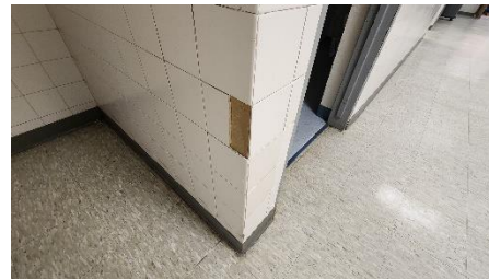
MISSING WALL FINISHES
