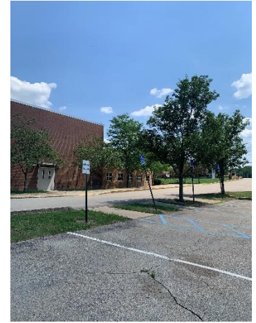
CRACKED ASPHALT IN PARKING LOT
