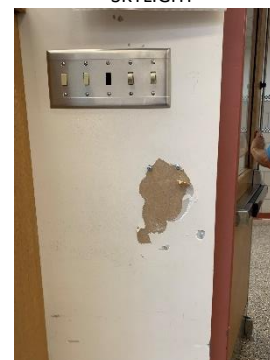
DAMAGED WALL FINISHES
