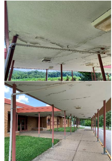
IMPROPER DRAINAGE AND PEELING PAINT AT BOTH CANOPIES
