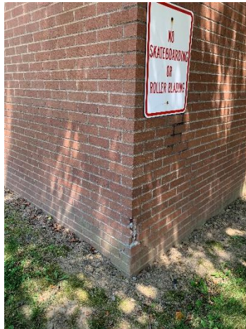
MISC. BROKEN EXTERIOR BRICK VENEER
