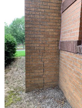
WALL CRACKING
