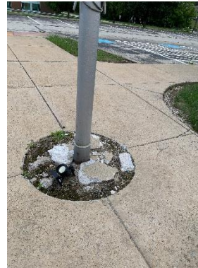
DETERIORATED PAVING
