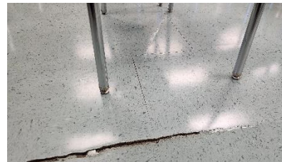
CRACK IN CLASSROOM FLOOR
