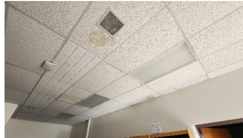
WATER STAINING AT HVAC SYSTEMS
