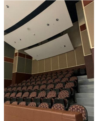
EXISTING WALL AND CEILING ACOUSTIC TREATMENT
