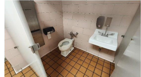
NO VERTICAL GRAB BARS AND NONCOMPLIANT CONFIGURATION
