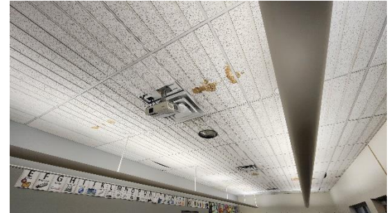
WATER STAINS NEAR HVAC UNITS
