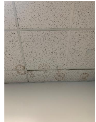
WATER-STAINED CEILING TILES
