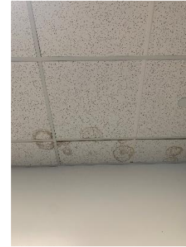
WATER STAINING AT HVAC SYSTEMS
