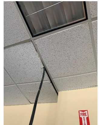
WIRES PROTRUDING FROM CEILING TILES
