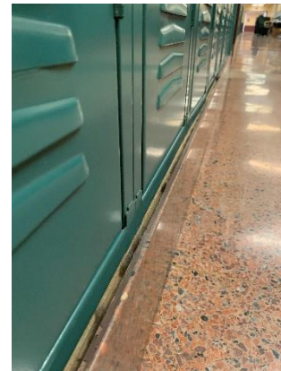
FINISHES PULLING AWAY FROM WALLS
