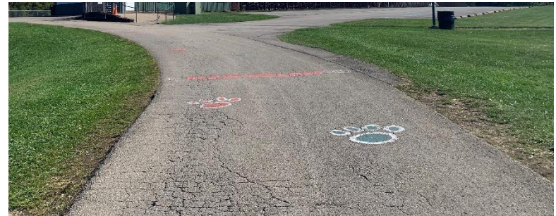
CRACKING PRESENT FROM HEAVY MACHINE USE. PRESENT THROUGHOUT SITE
