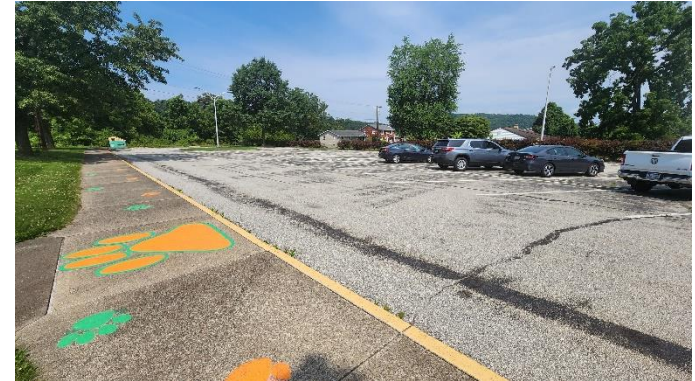
CRACKS IN ASPHALT AND CONCRETE AT FACULTY LOT
