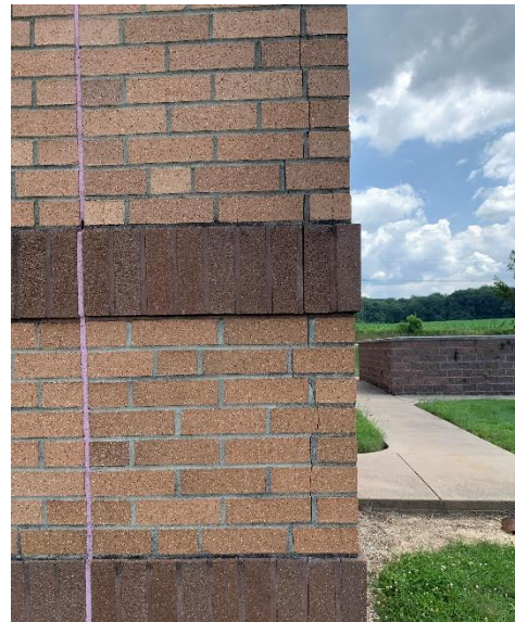
MASONRY CRACKING/ MORTAR DETERIORATION
