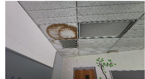
WATER STAINING AT HVAC SYSTEMS
