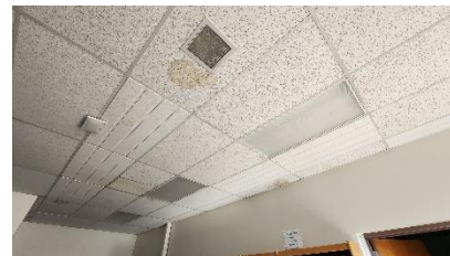
WATER STAINING AT HVAC SYSTEMS
