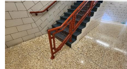
NON-COMPLIANT GUARDRAILS
