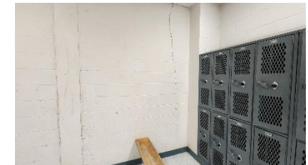
INTERIOR WALL CRACKS
