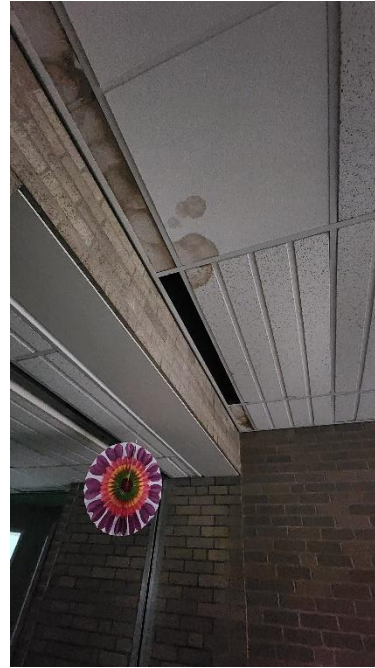
WATER STAINS WHERE ADDITION MEETS ORIGINAL BUILDING
