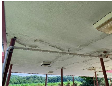
DETERIORATED CANOPY
