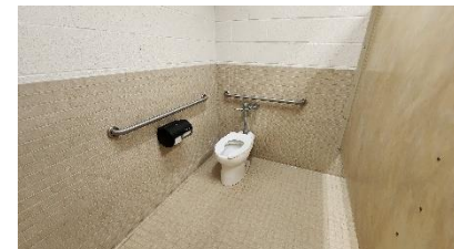
MISSING VERTICAL GRAB BAR
