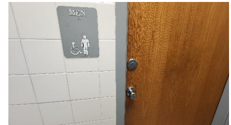
NON – ADA COMPLIANT DOOR HARDWARE
