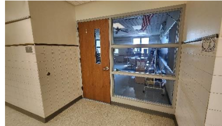
SIDELIGHT UPGRADED WITH IMPACT FILM
