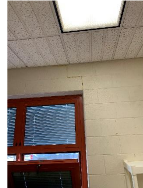
INTERIOR STEP CRACK
