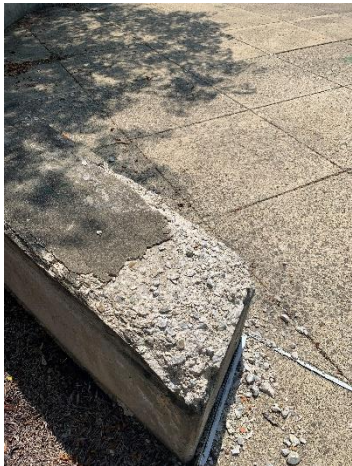
DETERIORATING CONCRETE AT ENTRANCE
