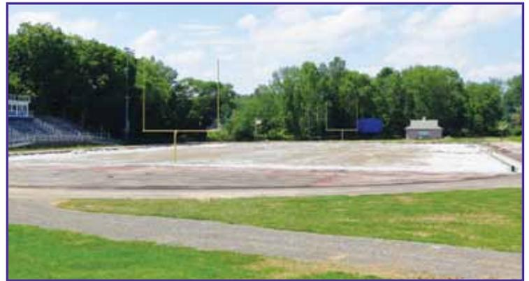
1996, and its rubber layer significantly deteriorated over time and is being replaced with 1.5 inches of asphalt. It will be repaved with new asphalt and rubber material, in addition to undergoing some necessary subsurface repairs.
