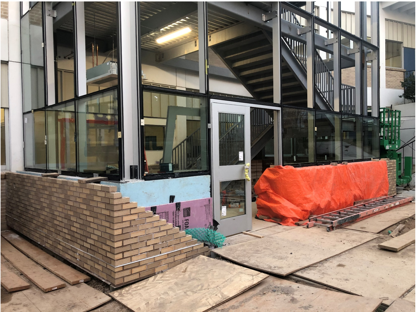
Week 35 – Progress of work for brick base & glass panel installation for Stair Tower
