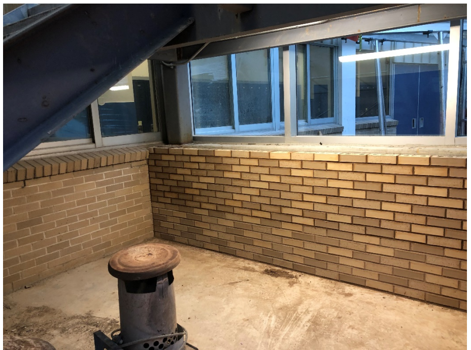
Week 36 – Interior brick finish to match the existing inside the Tower on the ground floor
