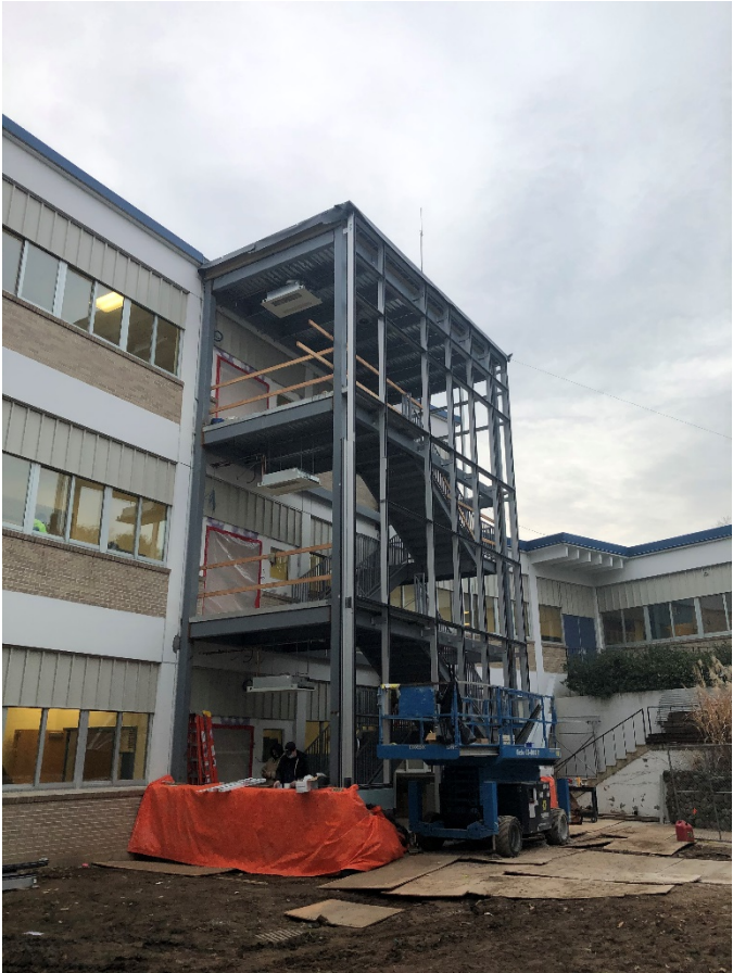
Week 34 – Mullions for curtainwall need to be installed on one side
