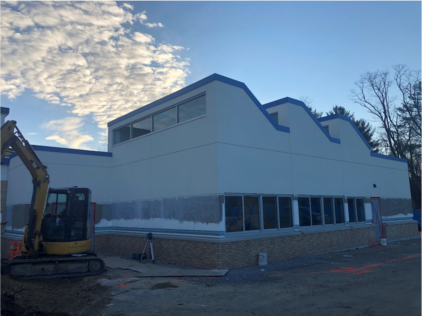
Week 33 – Edge flashing for roof for Art Room addition completed
