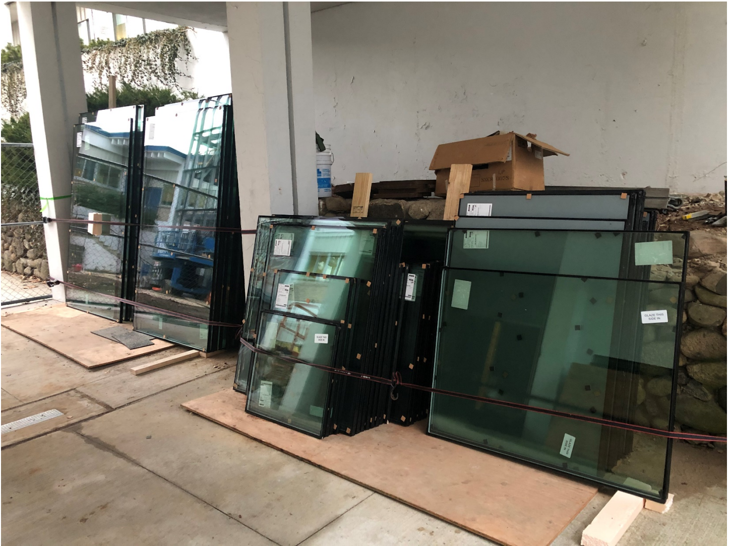
Week 34 – Glass units on site & ready to be installed for Stair Tower
