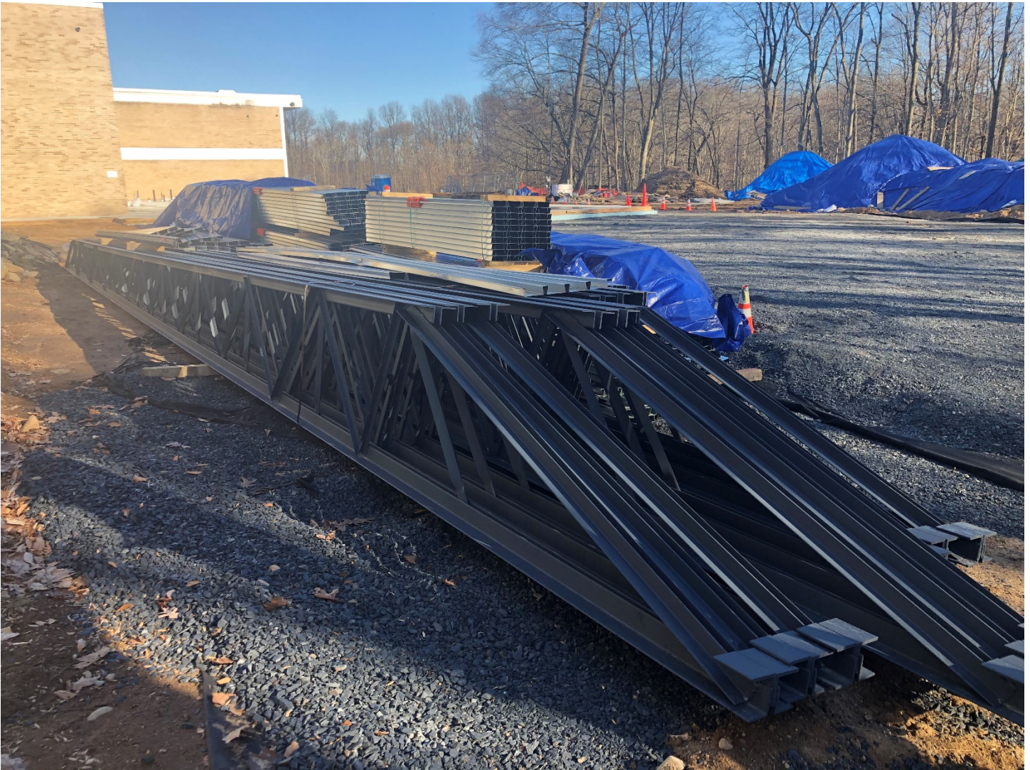
Week 33 – Steel trusses for Gym addition on site
