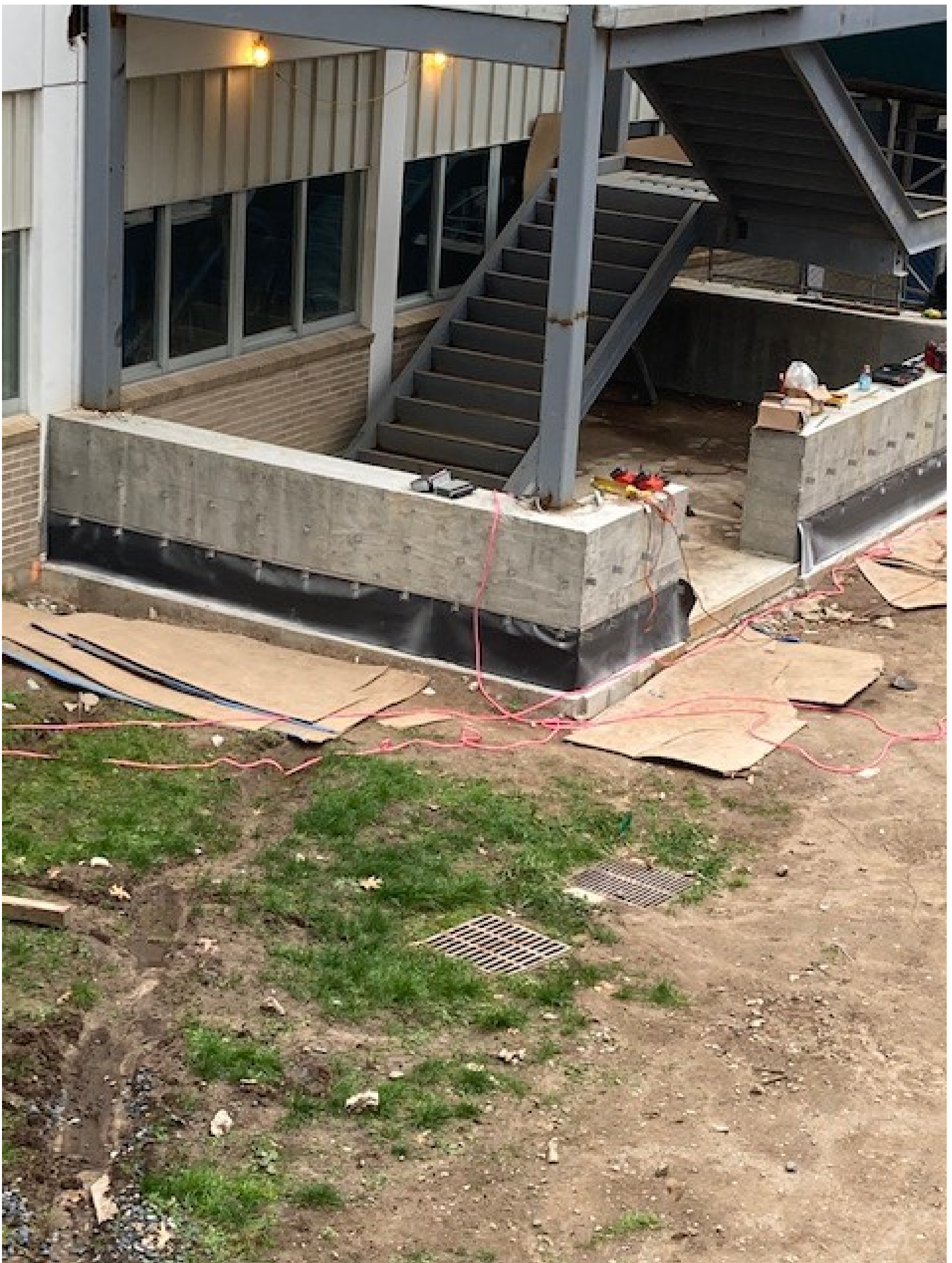
Week 29 – Beginning to prepare for the installation of the brick base for the Stair Tower
