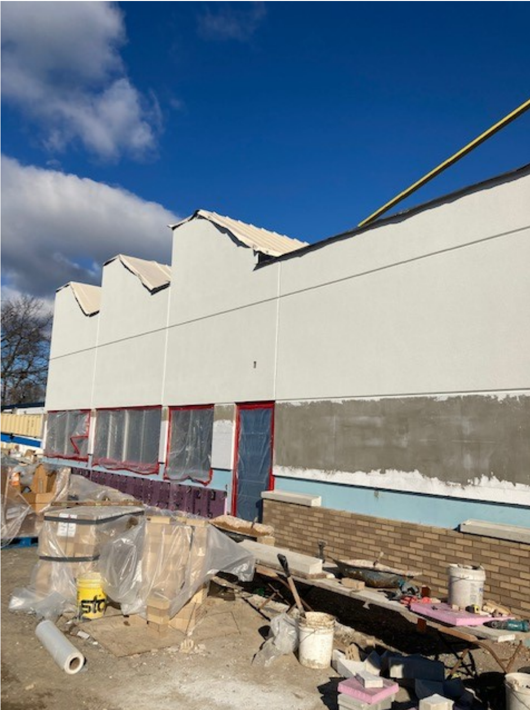
Week 29 – Brick work in progress with partial install of capstone trim for transition to EFIS
