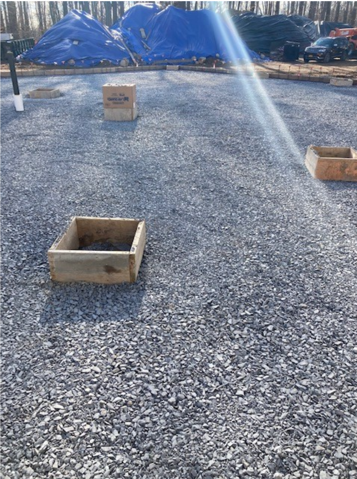
Week 29 – Gravel base spread out over the soil subbase and being prepared for the pouring of the concrete slab at the Music Wing for the end of the week & beginning of next week
