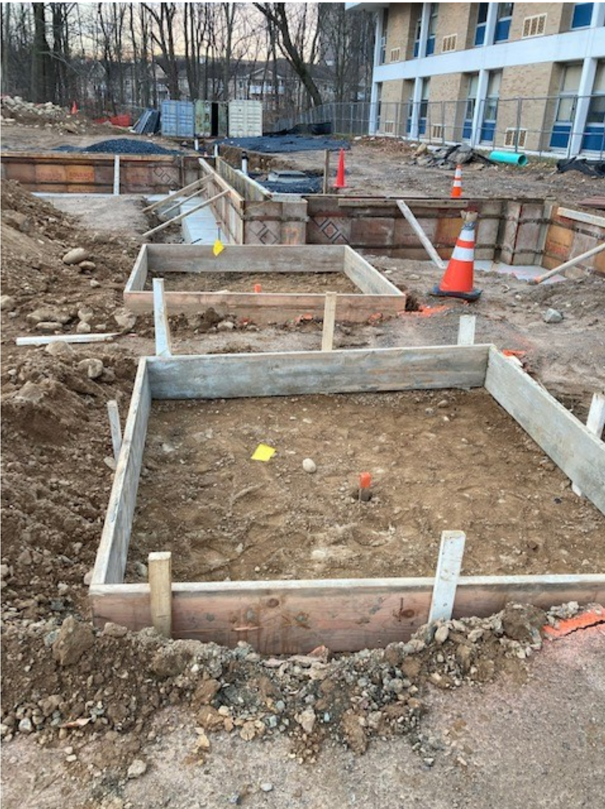
Week 28 – Concrete footings for Music Wing addition are completed, formwork going in for foundation walls & column footings
