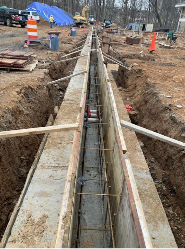
Week 29 – Rebar & formwork in place for pouring of the concrete foundation walls for the Music Wing at the beginning of the week
