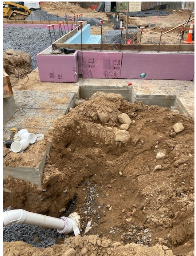
Week 29 – Foundation walls at Music Wing are completed with rigid insulation applied to the inner side & moisture barrier on the exterior and doing underground plumbing work mid-week
