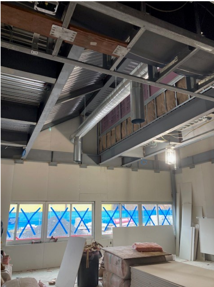
Week 29 – Gypsum Wall Board installation along with exposed steel structure & ductwork
