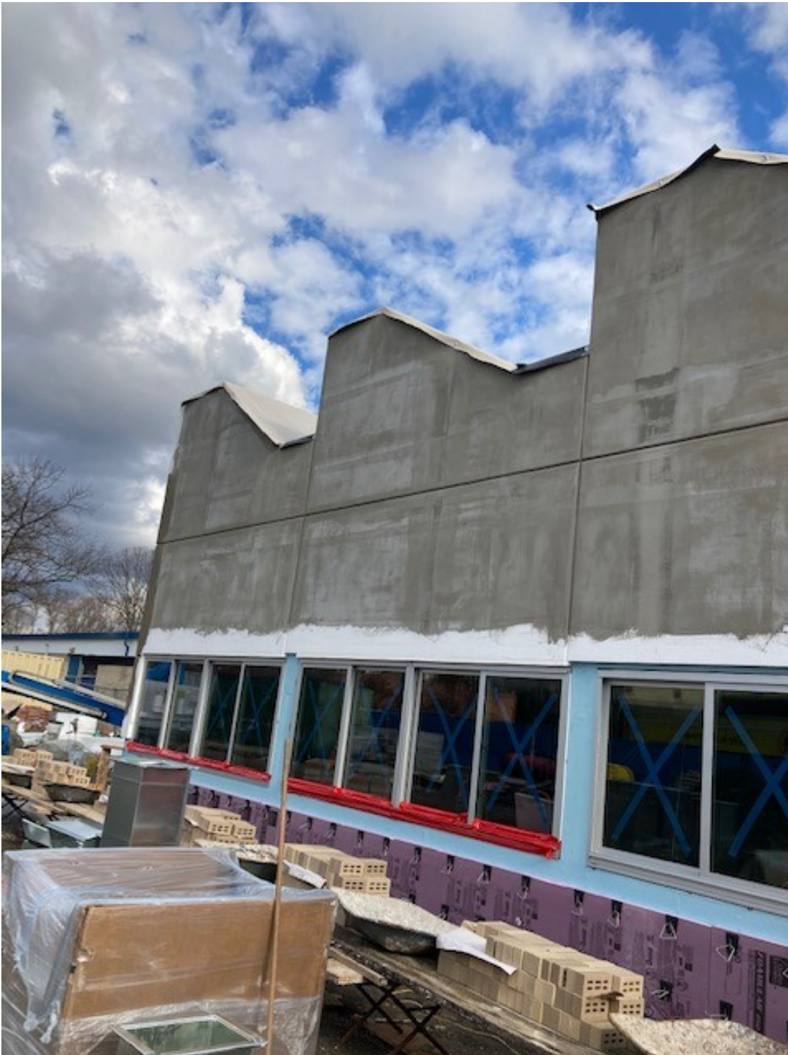
Week 28 – Windows installed & EFIS cladding in progress for Art Room addition
