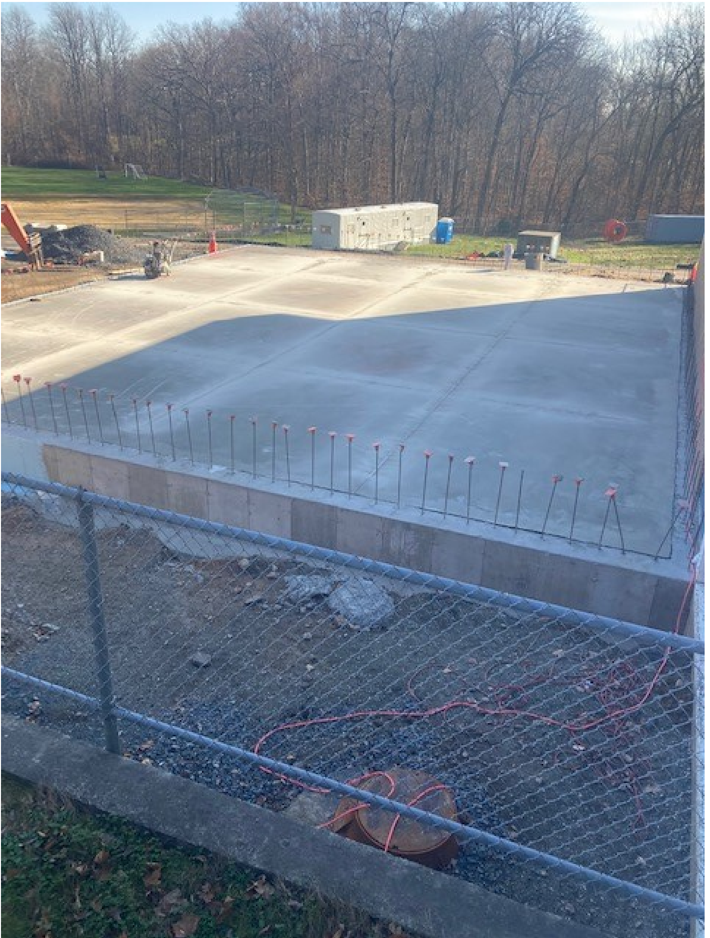
Week 28 – Concrete slab for Gym addition poured
