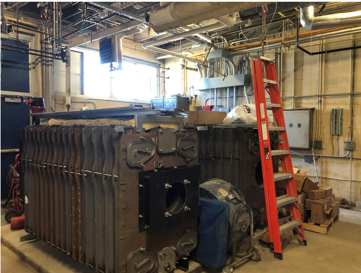
Week 20 – New Boilers being installed
