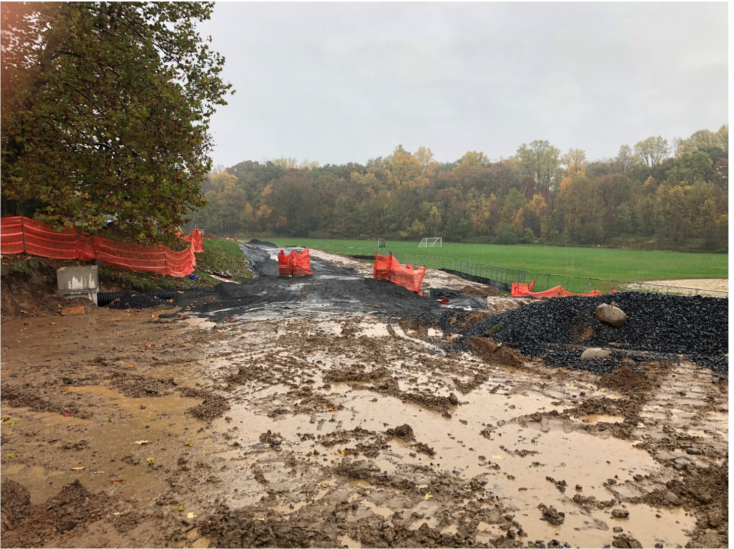
Week 23 – Progress of the work for the access road along with some drainage structures in place (wrapped by the orange safety fencing)
