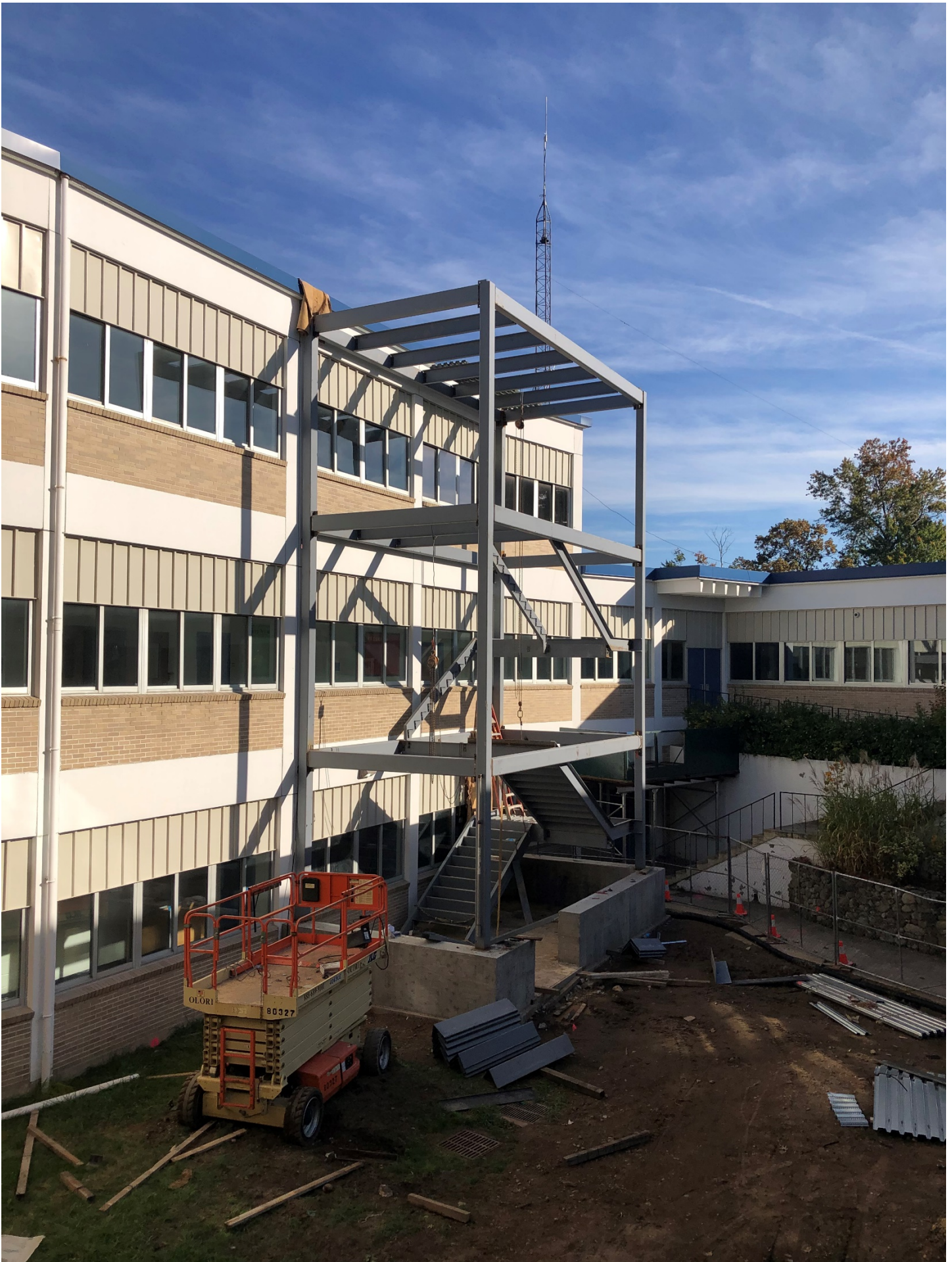
Week 21 – Structural steel framing completed and stairs being erected for the Stair Tower
