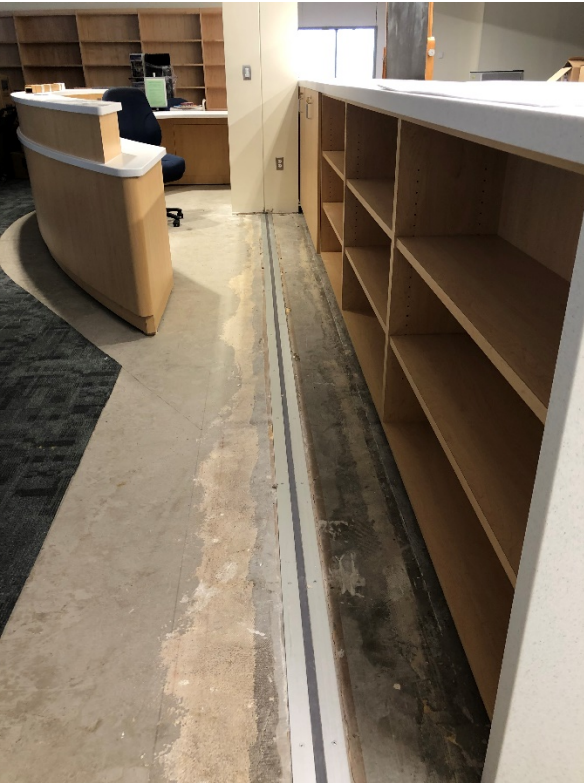
Week 20 – Installation of the expansion joint assembly completed in the Library
