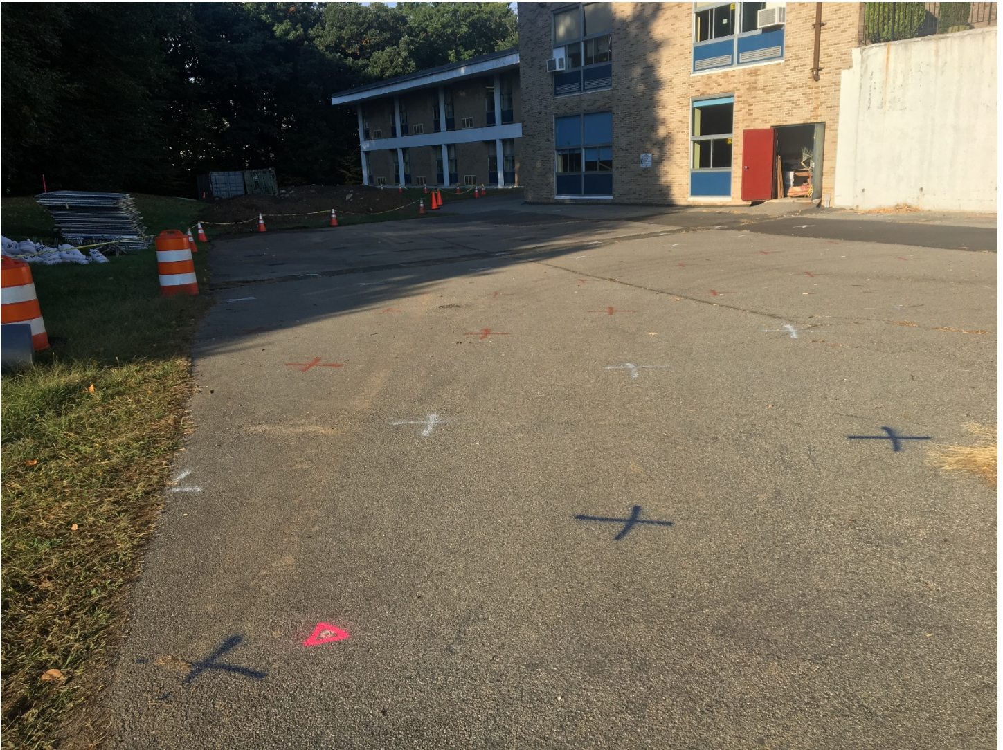
Week 19 – Mobilization of the site with some markouts for existing underground utilities on the pavement
