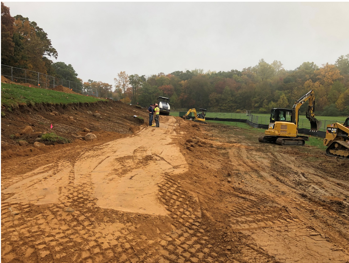
Week 22 – Cutting and filling site for proposed access road
