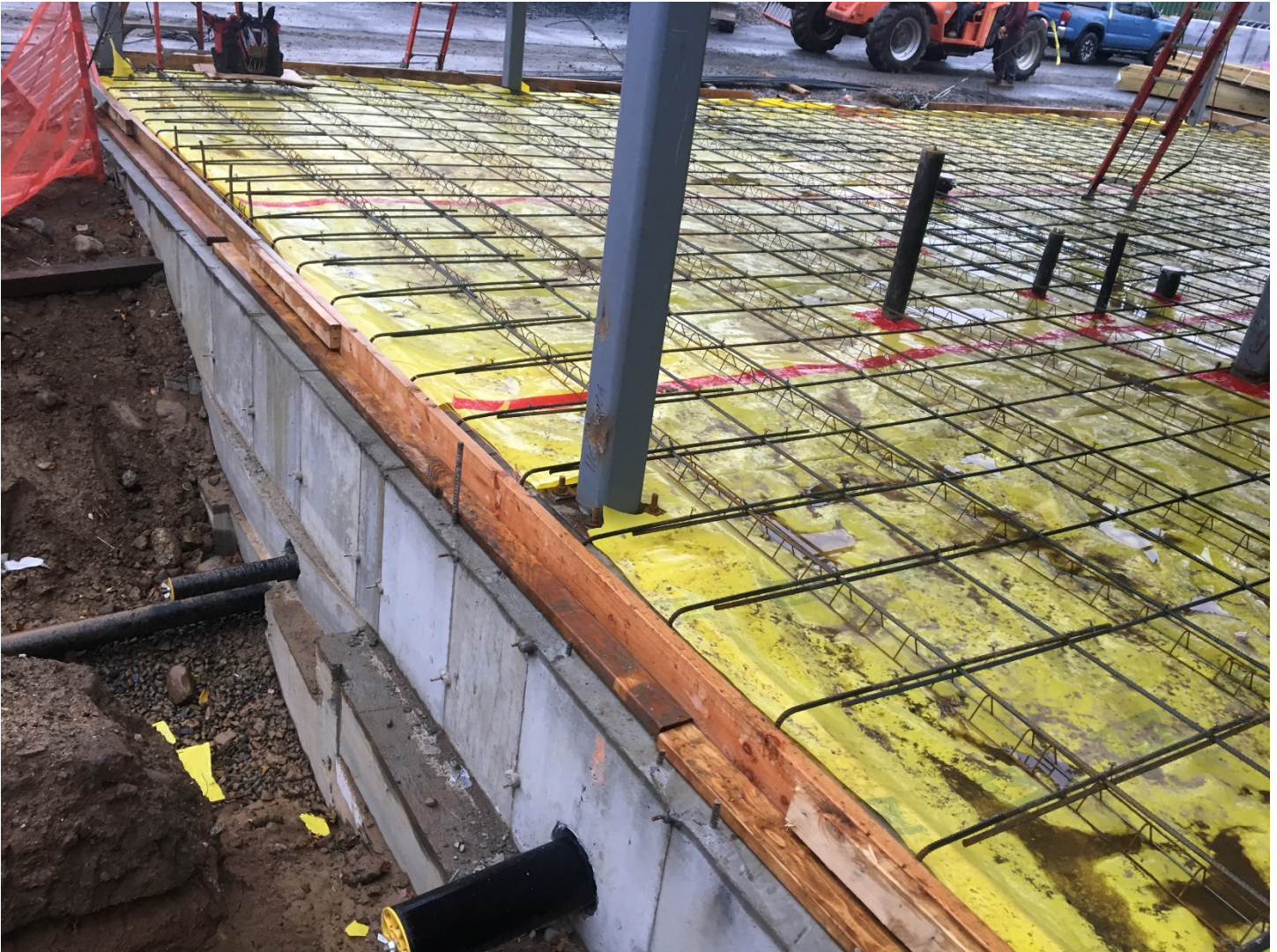
Week 19 – Preparation and setup for the pouring of the concrete slab for the Art Room addition next week
