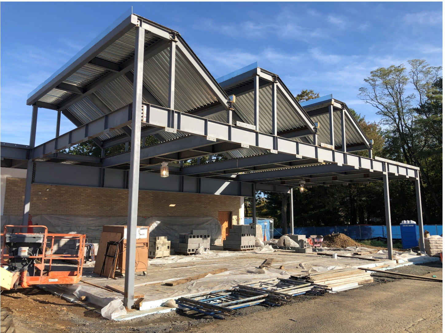
Week 21 – Metal deck installed on roof, wood blocking for roofing started and CMU block wall along the existing building has begun
