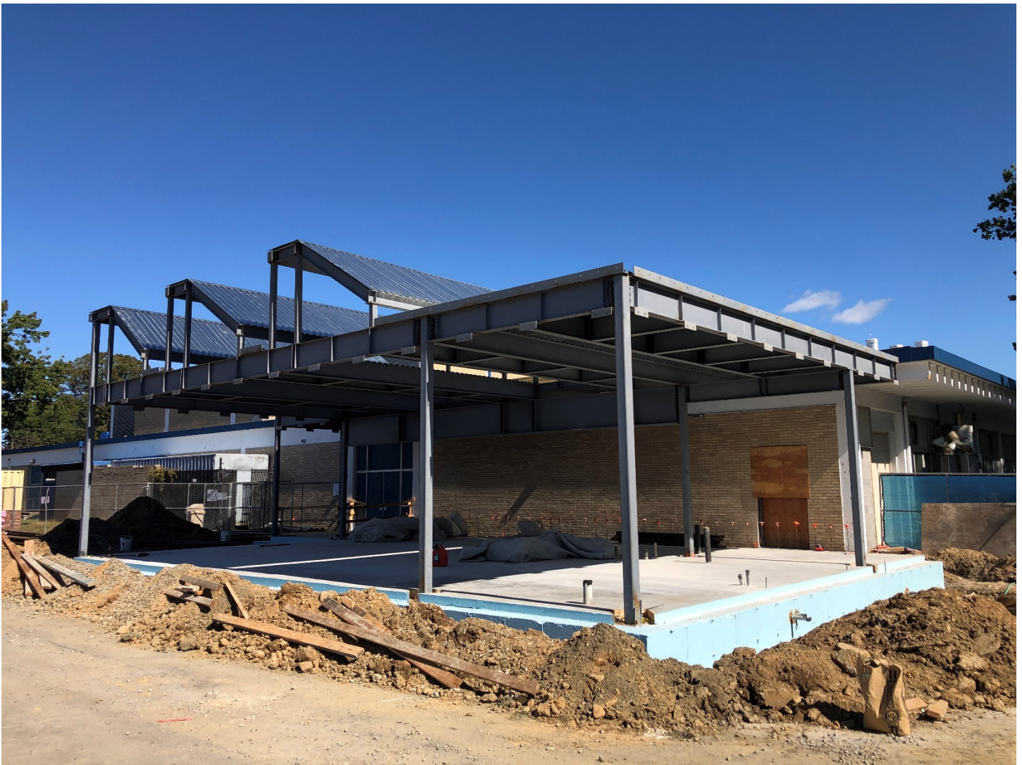
Week 20 – Structural steel work completed for Art Room addition
