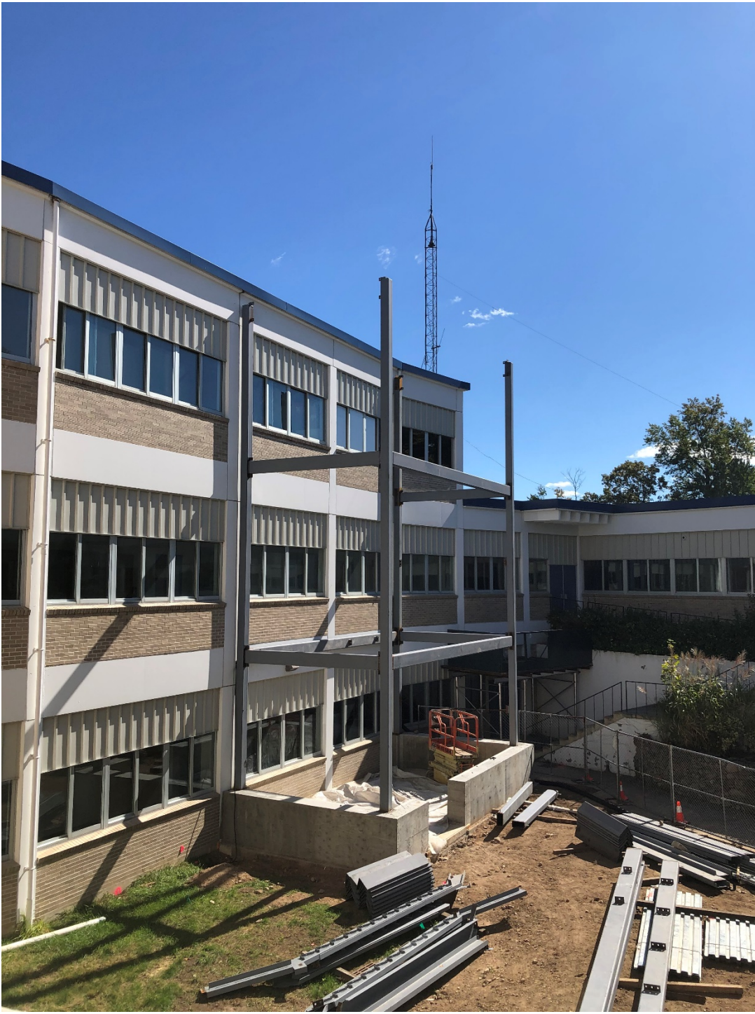
Week 20 – Structural steel being erected for the Stair Tower
