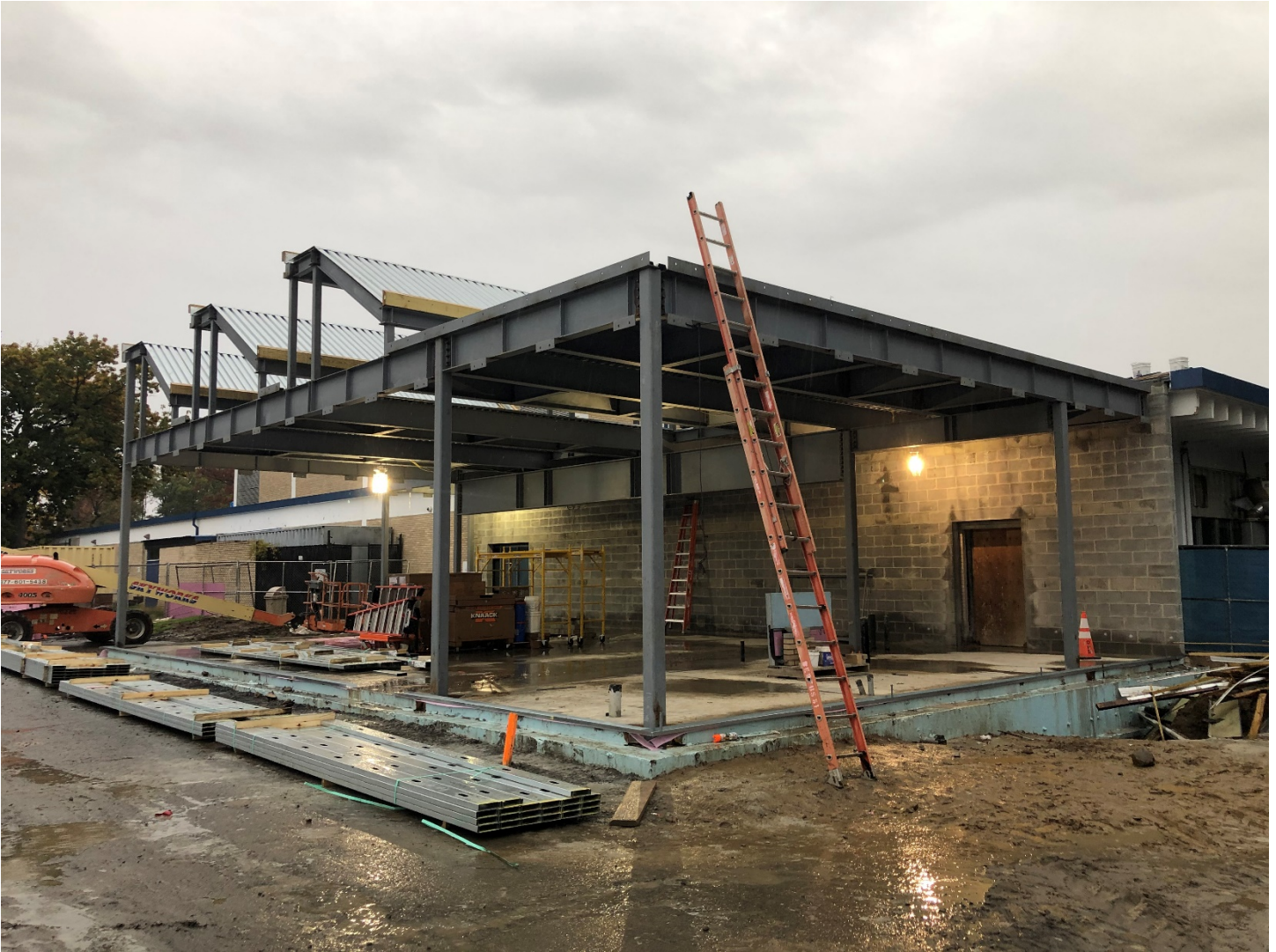
Week 23 –CMU block wall along the existing building finished at the Art Room addition
