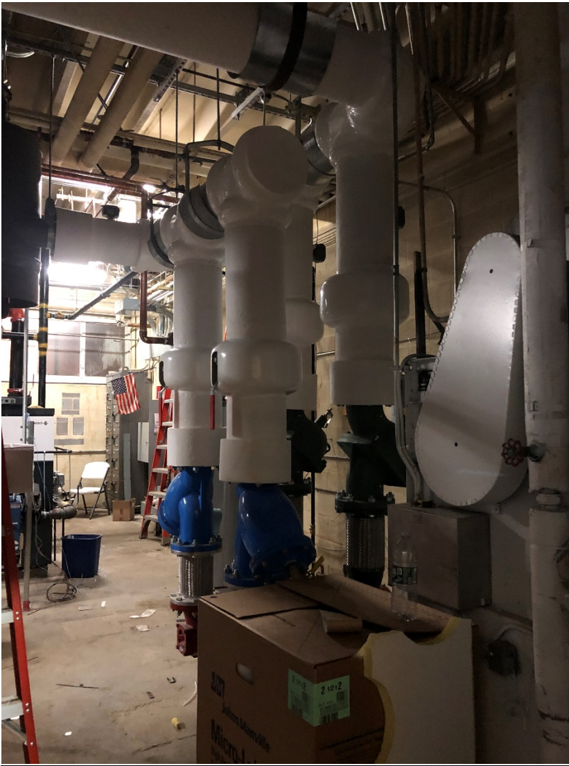
Week 22 – Piping in Boiler Room being insulated
