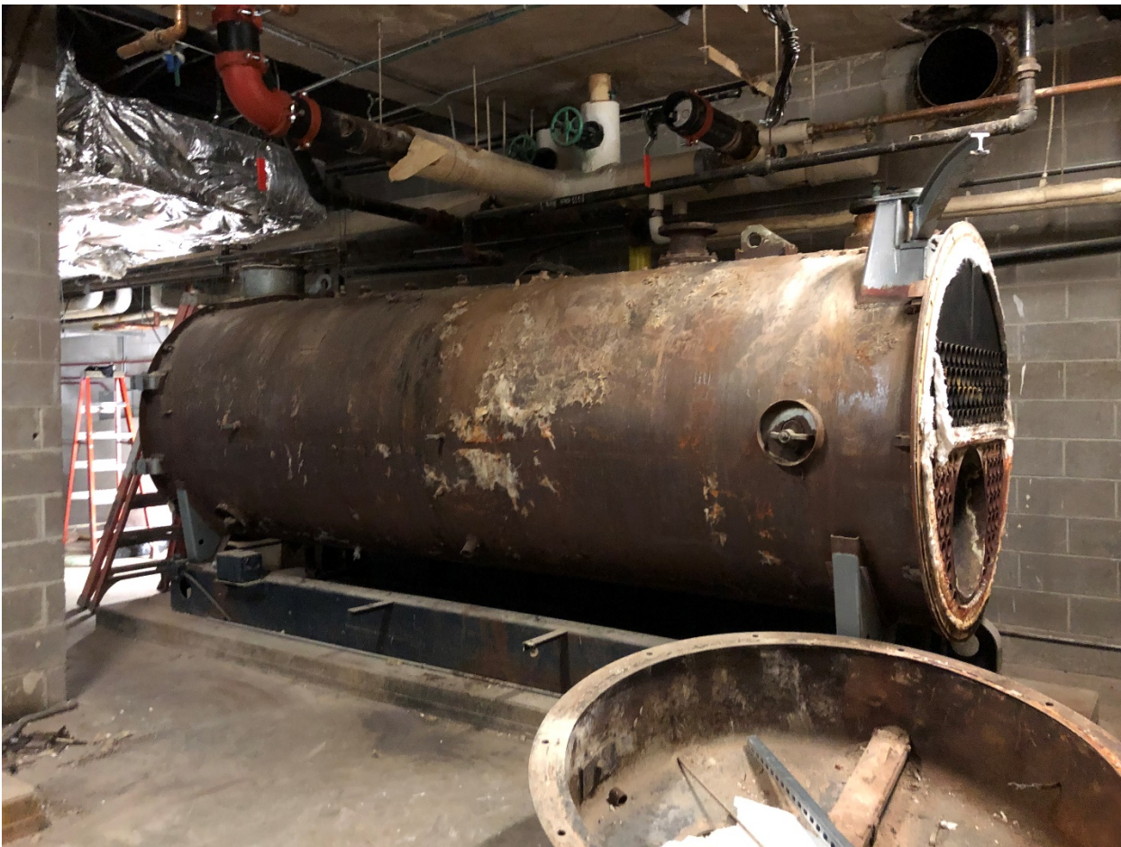
Week 20 – Old boiler in the process of being dismantled for removal
