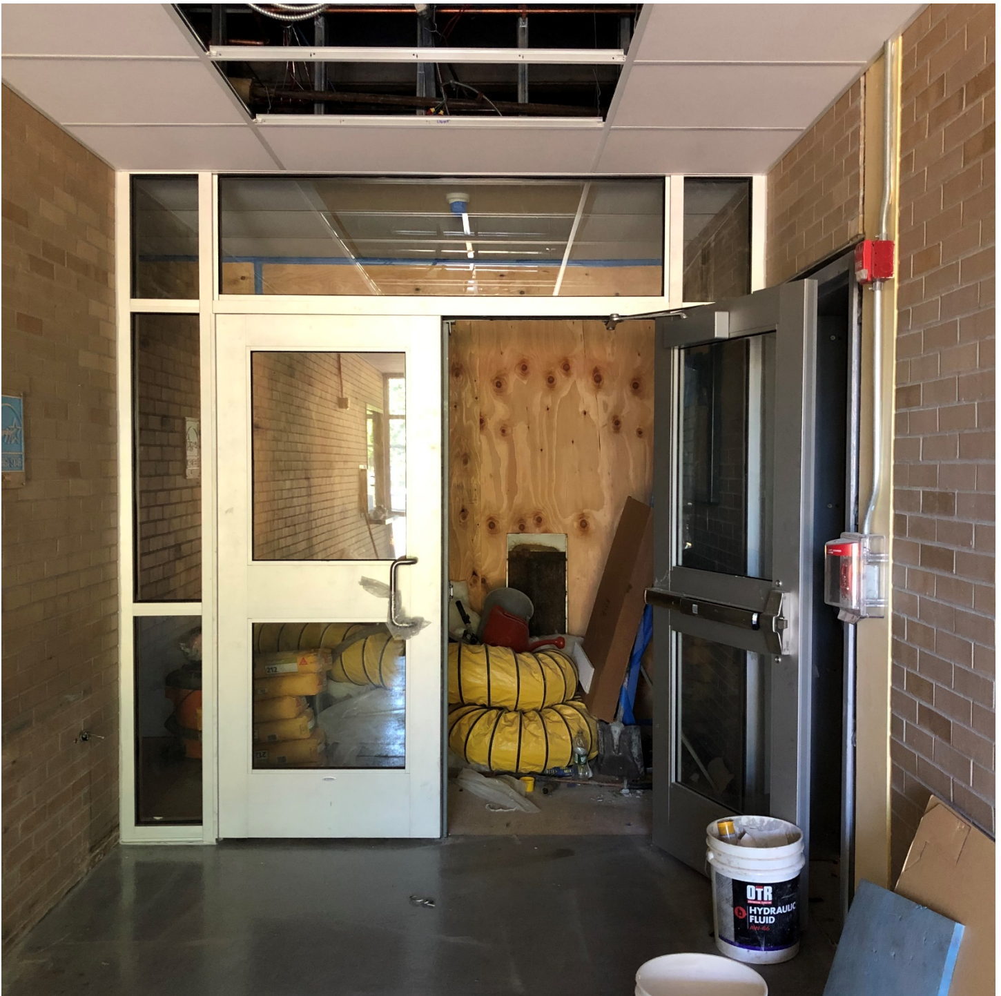
Week 20 – Inner Storefront Doors installed for the Security Vestibule
