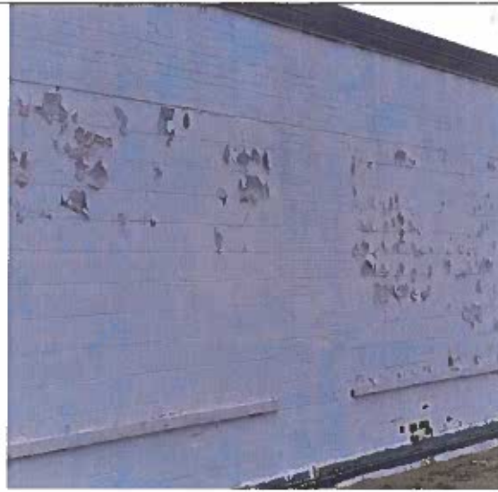
Upper Gym wall-CMU block, leaking needs significant repair
