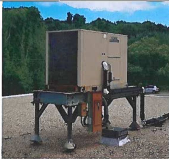
Stage Roof Top Unit, out of commission, should be removed
