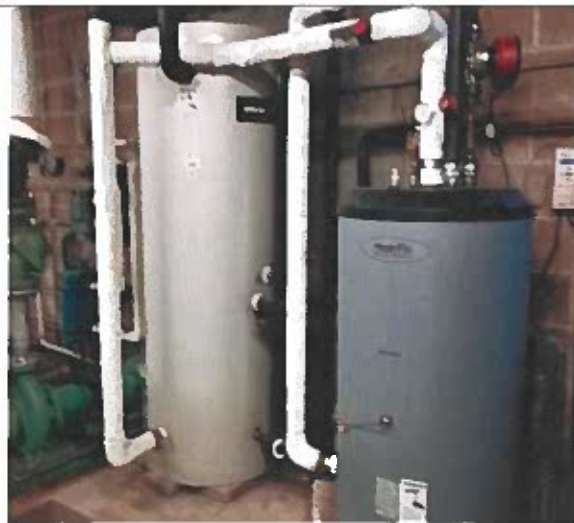
Solar tank with newer High Efficiency domestic Hot Water tank 100 gal. capacity, (good condition)
