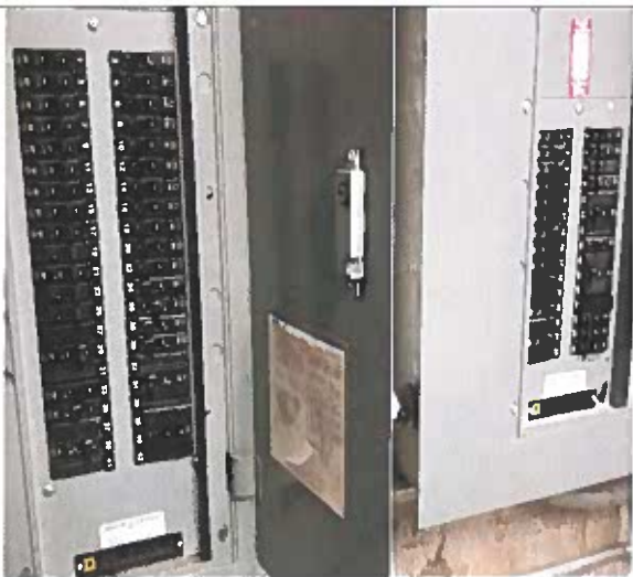
Two of three electrical panels with room for future circuits
