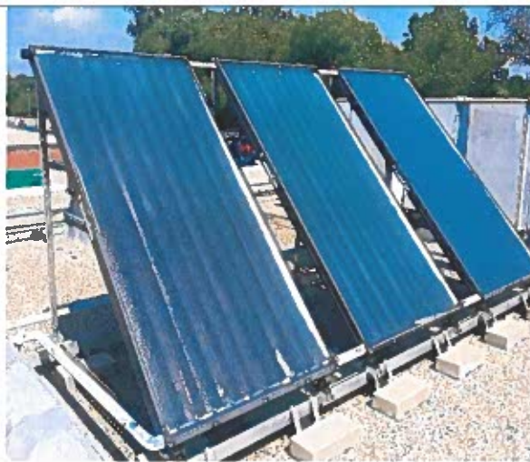
Thermal hot water panels Good Condition
