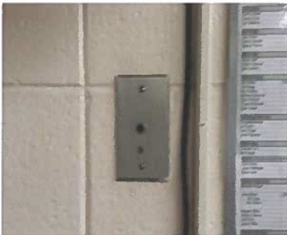
Thermostat plate sensor in each Classroom
