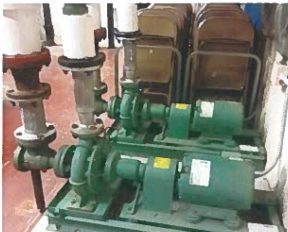
Water Circulating Pumps
