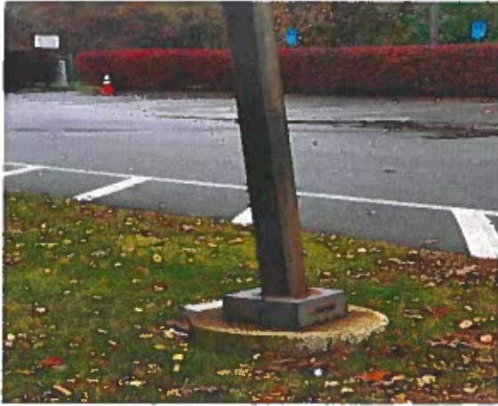
Light Pole with rusted base, recommend replacement
