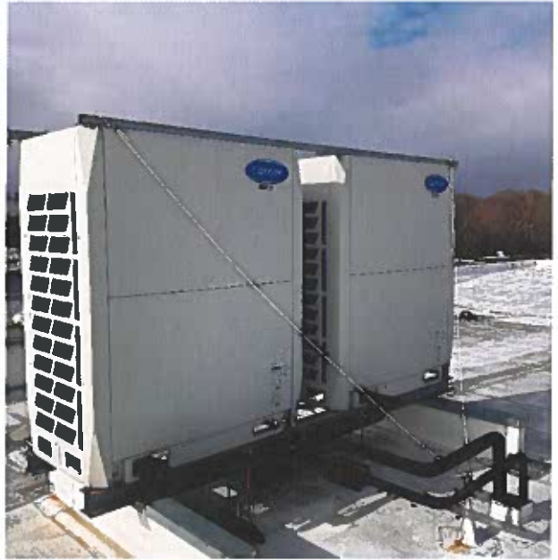
2 of 4 Carrier units for 2 nd floor AC
