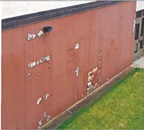
Exterior CMU wall (Maintenance required)
