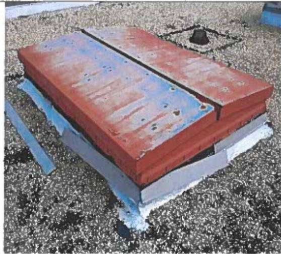
Flashing of the 3-auditorium smoke hatches, needs to be addressed
