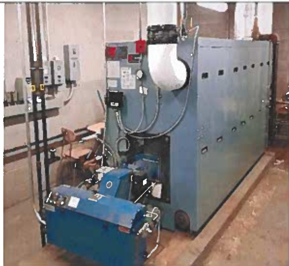
Newer Boiler (1 of 2) with Power Flame burner (good condition)
