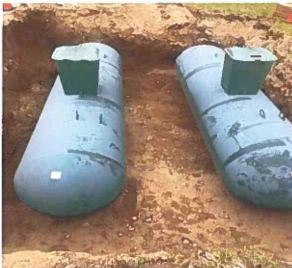
Two new underground propane tanks
