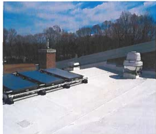
Roof with hot water solar panels
