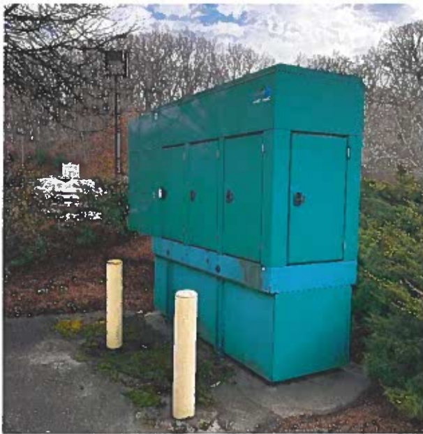
100 kW Generator with diesel tank
