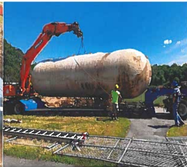
20,000 gallon tank removal
