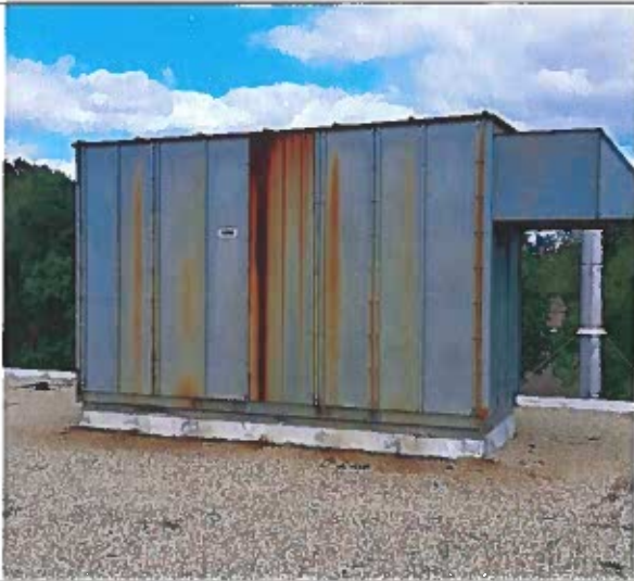
Practice Gym RTU Typical condition of most units (29 years old)
