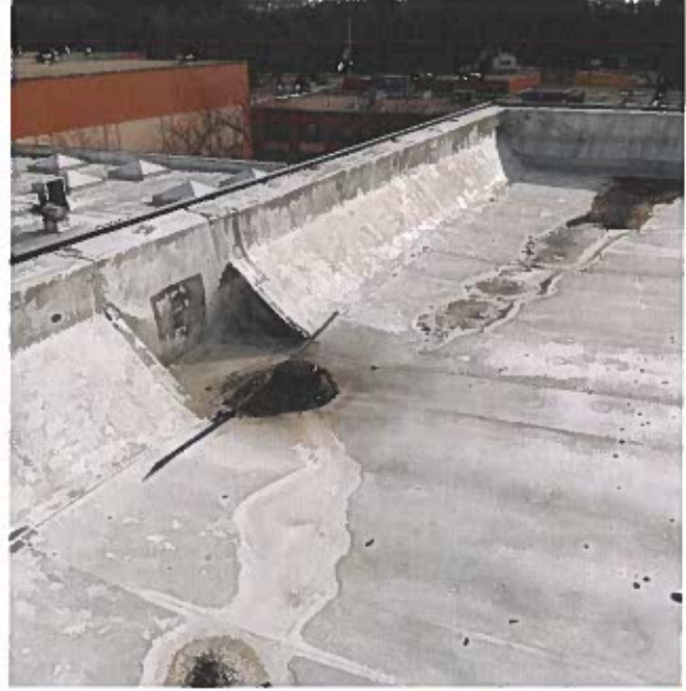
Roof drain and ponding
