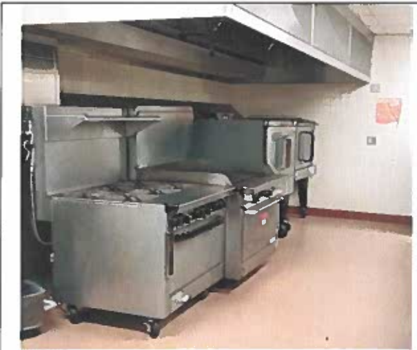
Original exhaust hood (Poor Condition)
